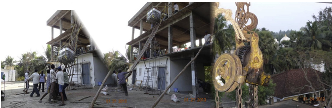
Fig. 22. Because there are no industrial cranes present in this remote village in India, old-fashioned ingenuity through the use of cut tree-poles was used to lift the 1-ton water purifier up many stories to the water storage tanks previously placed there for gravity distribution. Because of the size of the pump, the unit needed to be placed on the same story in this isolated instance. Inch by inch, with the assistance of many school workers and much prayer, the unit was slid up the poles by the use of the auto-engine hoist ratchet. Finally, the unit is received with success.
