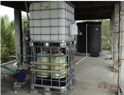
Fig. 20. A portable water purification unit is displayed here showing a compartmentalized unit, which is easy to install, requires only backwashing and no cartridges, exceeds US Environmental Clean Water Standards, and produces enough clean water for 6000 persons for over a 10-year lifespan (W.M.I. Portable Water Purification Unit).
